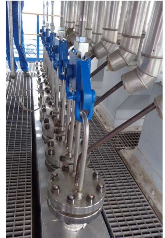
EARTH ® tubes in-tube thermocouples
